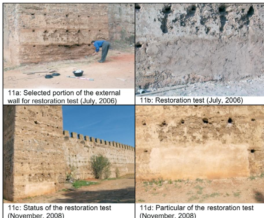
Fig. 11 - Documentation of the restoration test made on the external wall of the Chellah.
